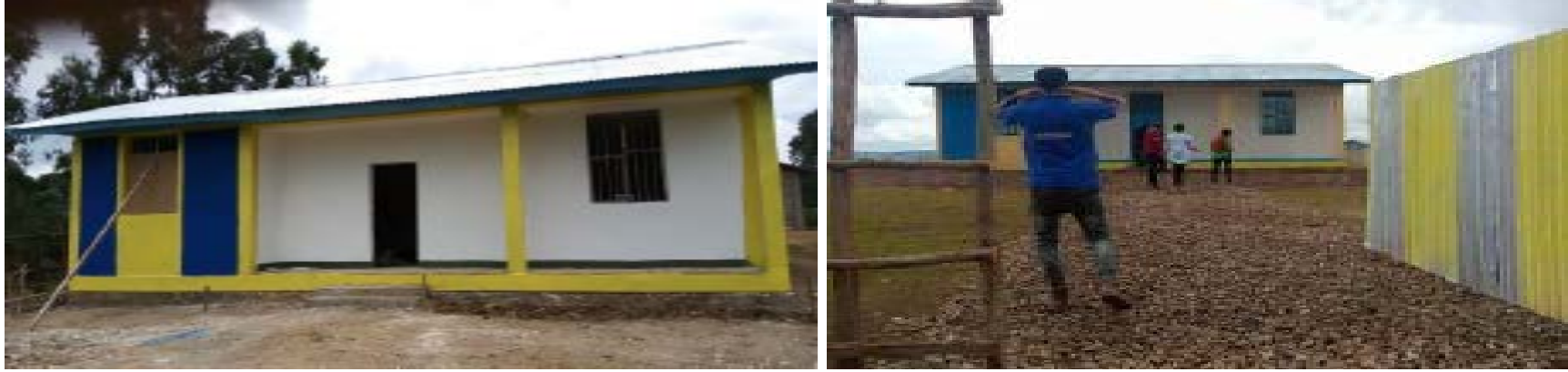
Health service is improved by construction of OPD blocks in West Guji (Hambela Wamena Woreda, Sika Bokosa Kebele) and Gedeo Zone (Gedeb Woreda Banko Tetetu Kebele )
