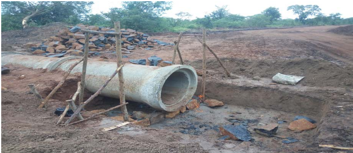
Culvert at Punido 1 camp
