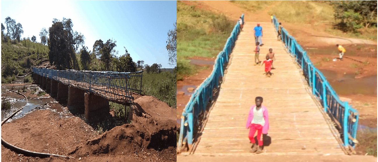
Wooden bridges in Gure-Shambola Refugee Camp
