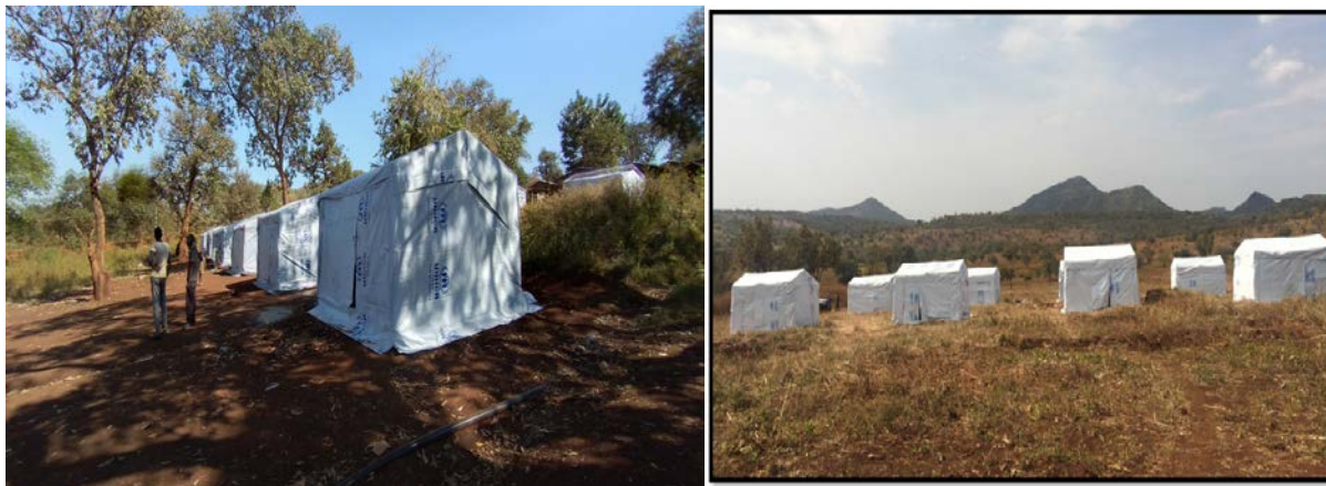
Emergency Shelter at Gure Shombolla and Tesore Refugee Camps
