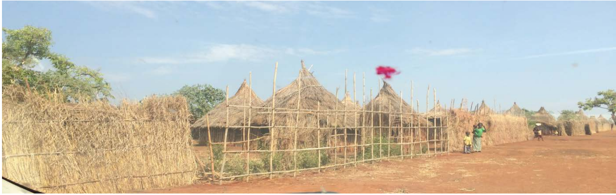
Transitional shelter Maintenance at Bambasi (Assosa)
