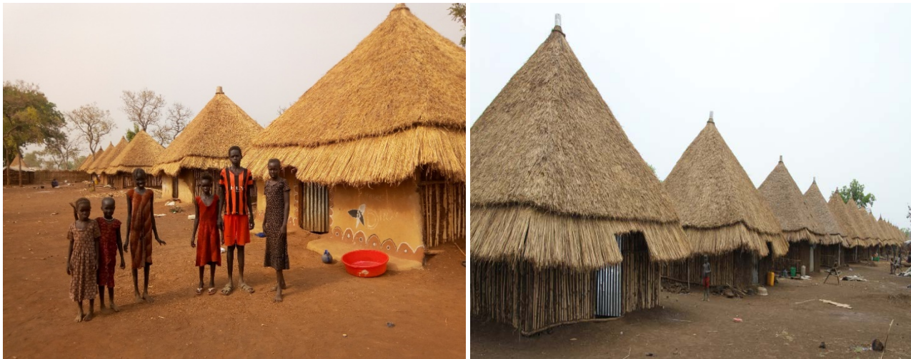
Transitional Shelter at Nguenyiel Refugee Camp
