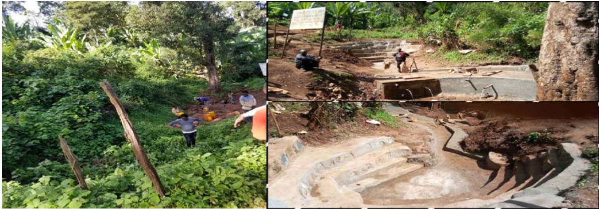
Sodu spring (Before Rehabilitation)
