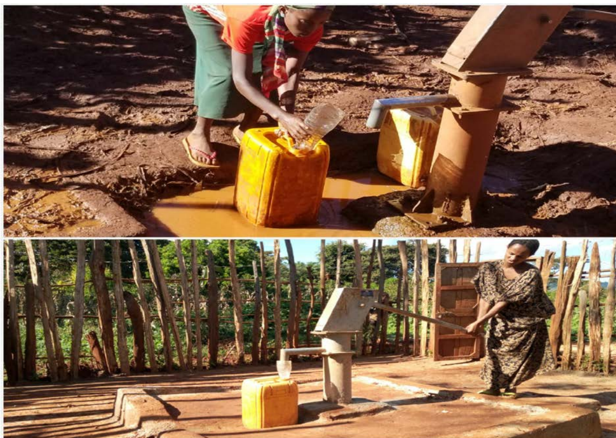
Meda Shallow Well before and after rehabilitation
