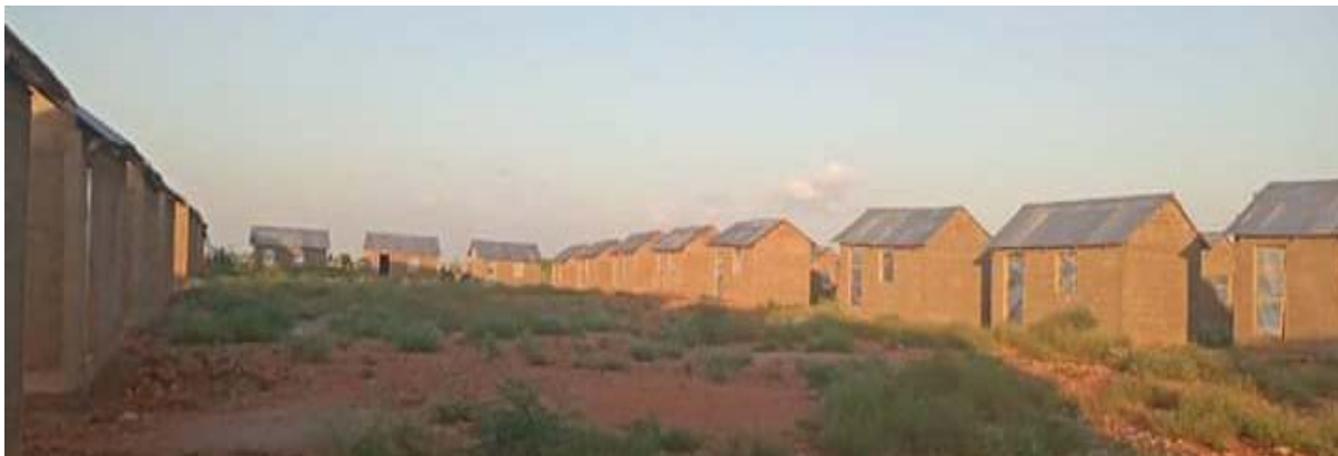
Improved Transitional Shelters at Buramino Camp
